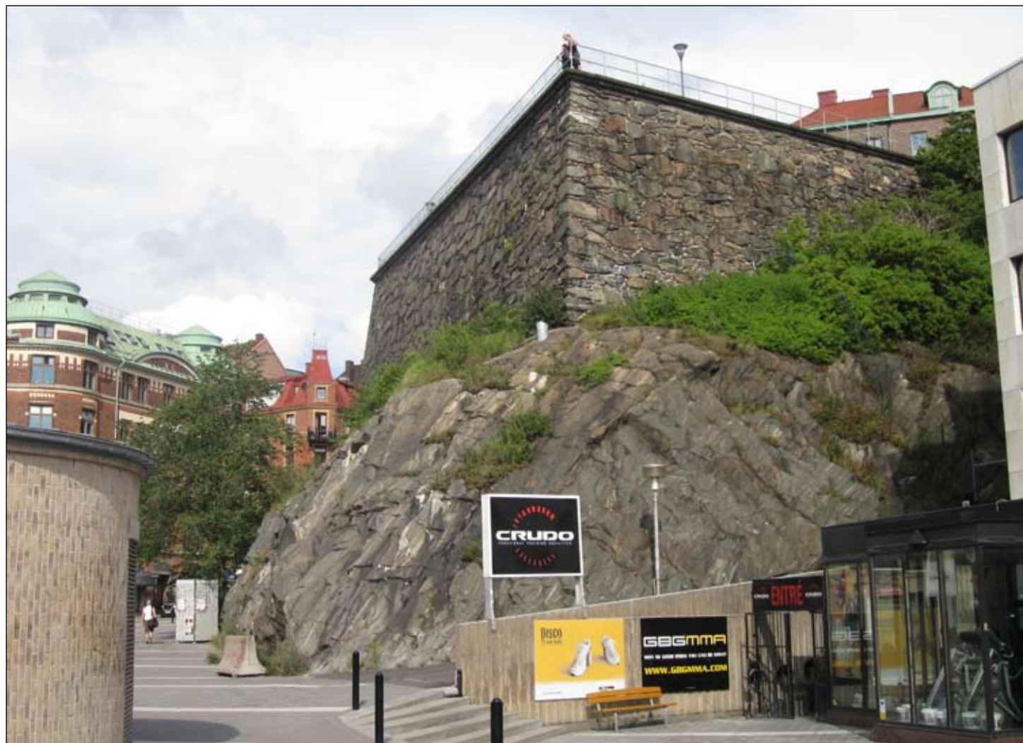
The only extant part of the old city wall in Gothenburg is at Charles Gate.
